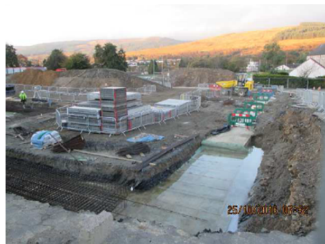
7 Sports Hall footprint following drainage works
