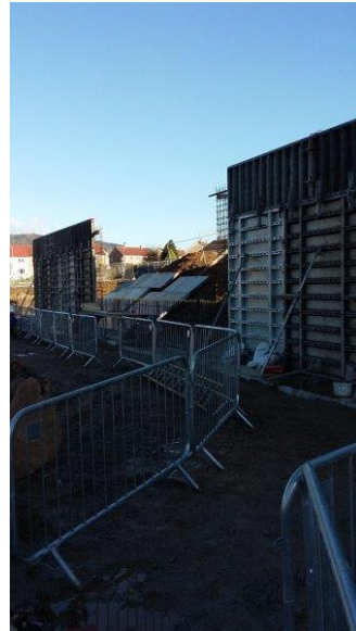
6 Erection of retaining wall
