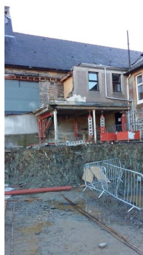
8 Additional structural support added to the rear of 1881 building
