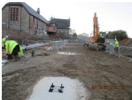
3 Classroom footprint following drainage works
