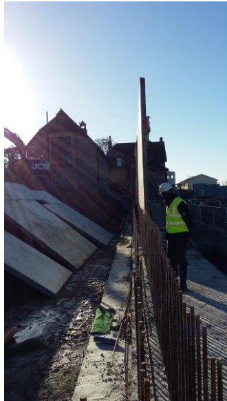
5 Reinforcement to the retaining wall
